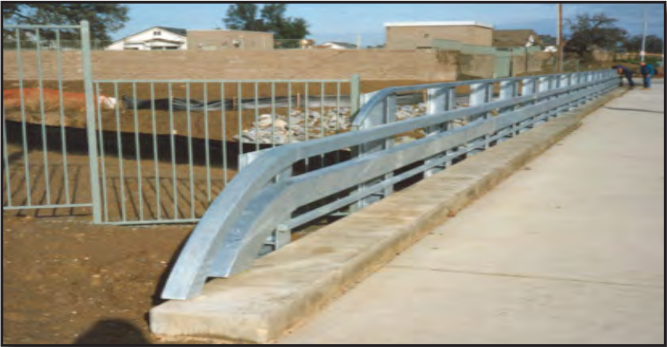
Typical Metal Tube Bridge Railing
