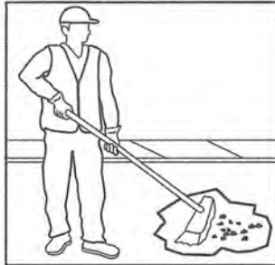
CLEAN SURFACE. Remove dust and debris with shovel or broom
