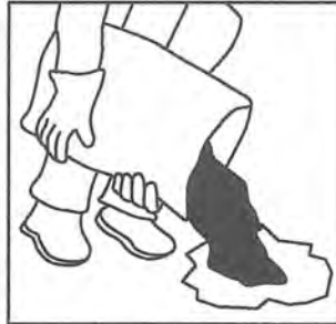
POUR POT HOLE PATCH. Overlap edges by 1" (2.5 cm); for potholes deeper than 2" (5 cm), apply in layers. Do not pour over clay, ice or mud. Dispose of bags properly.
